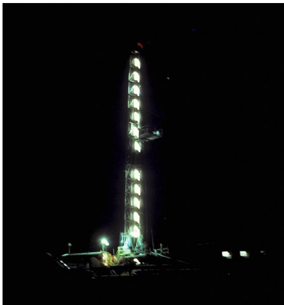
Gas drilling at night
